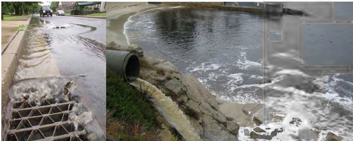
Traditional drainage management includes pipes and other grey infrastructure to get water away from buildings and roads. This leads to discharges of polluted water directly to oceans, lakes, and streams.
