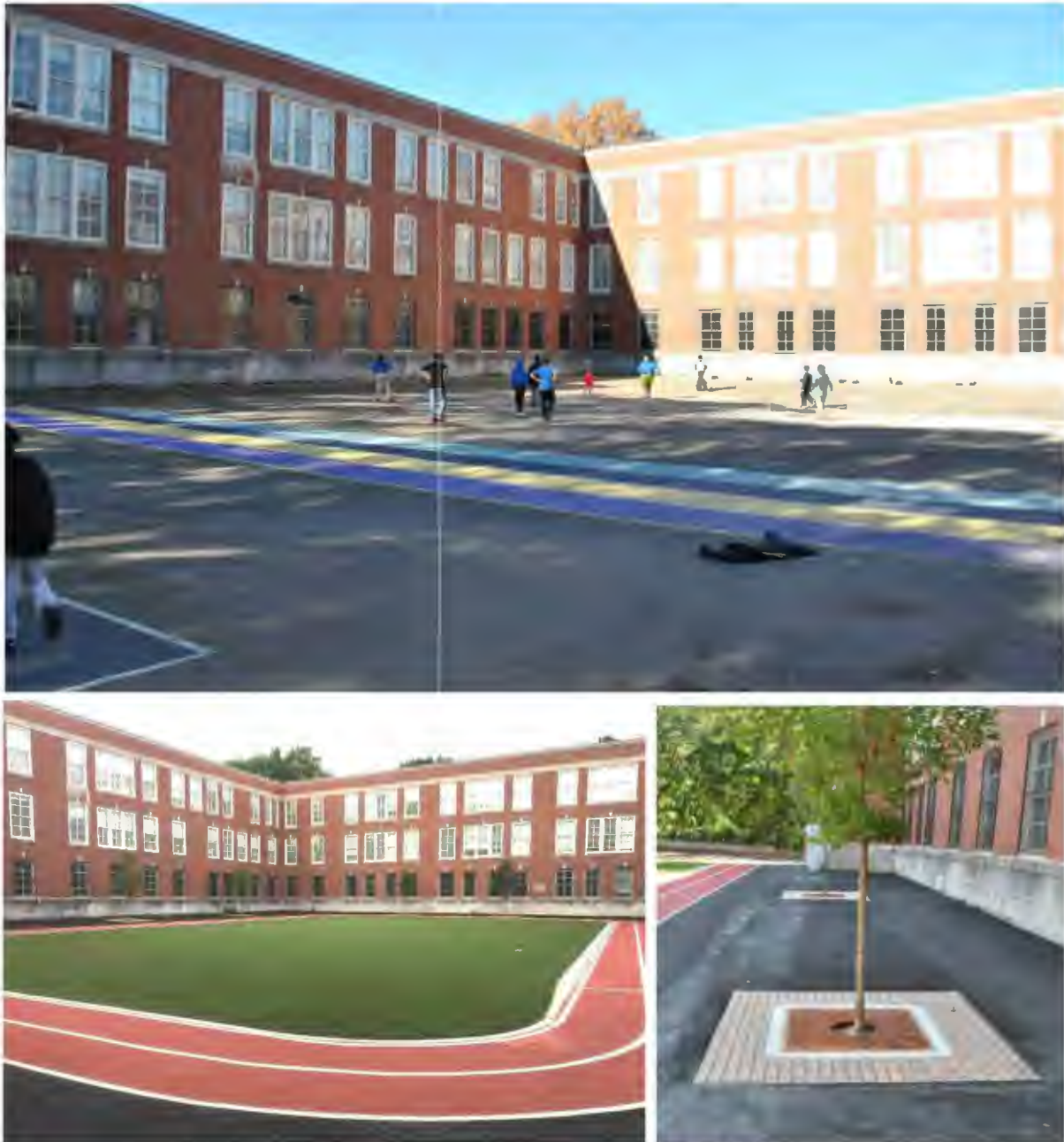
Figure 8. Before and after photos of the interior courtyard conversion to field with perimeter tree pits.
