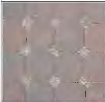
Porous paver, gravel fill
