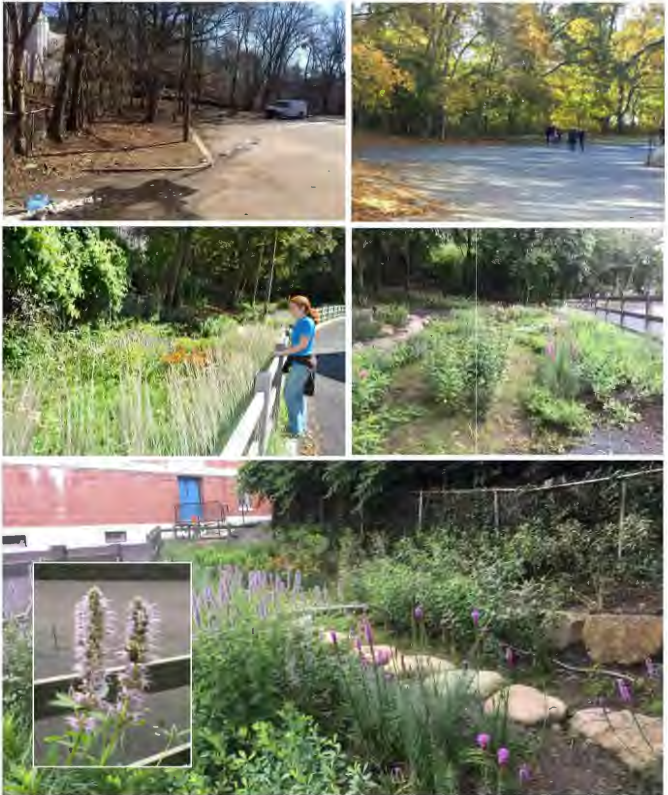
Figure 9. Before and after photos of the eastern corner conversion to bioretention.
