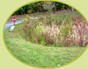
Constructed Stormwater Wetlands
