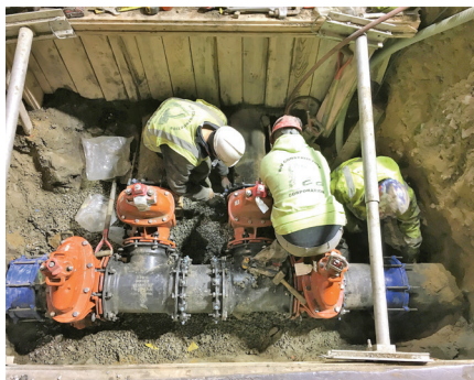
Installing water meters on Brookline Avenue.
