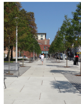
Residents stroll through Central Square in East Boston that feature permeable paver sidewalks designed to absorb rainwater.
