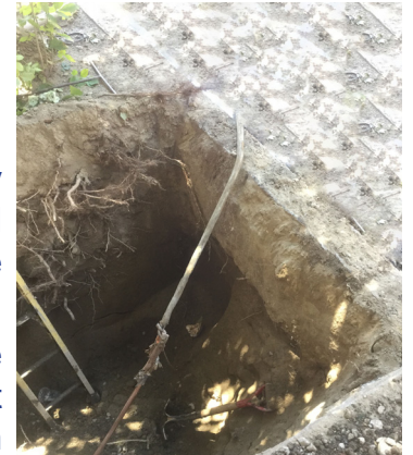
BWSC replaces lead lines through the Lead Incentive Replacement Program.
