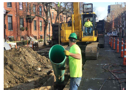
BWSC projects include improvements to sewer lines in the South End.
