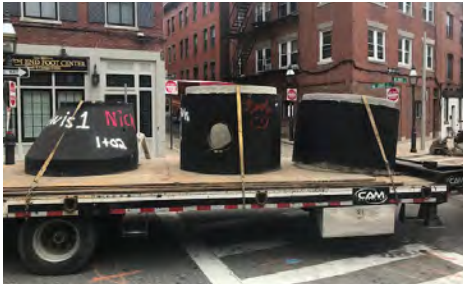
Catch Basins ready for installation
