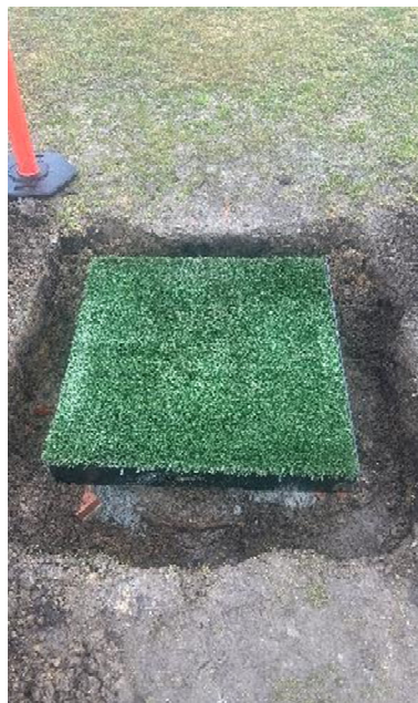
Buried manholes in Moakley Park are raised and fitted with turf covers in ballfields.
