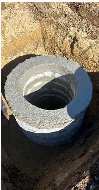
Buried manholes in Moakley Park are raised and fitted with turf covers in ballfields.
