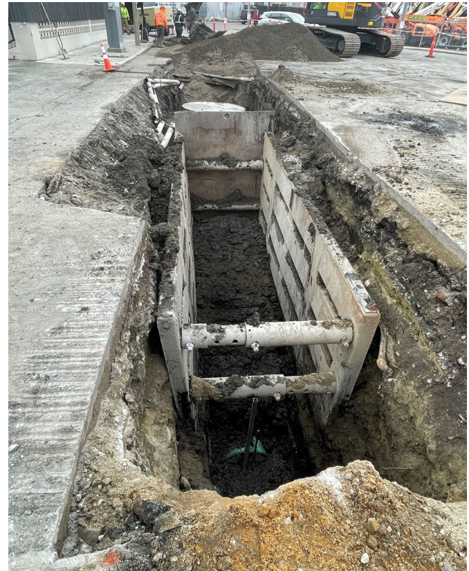
Sewer Trench on D Street
