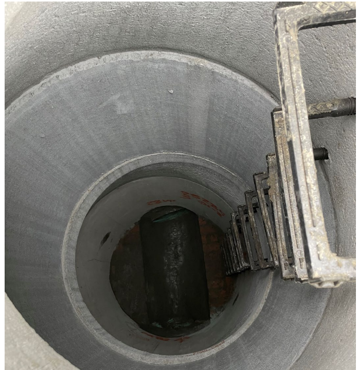
A view into a D Street sewer manhole.
