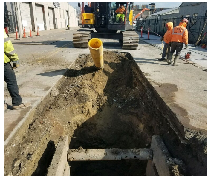
D Street sewer trench and abandoned gas pipe removal.
