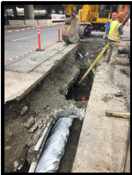
Installing Water Main Albany Street Near East Berkeley Street
