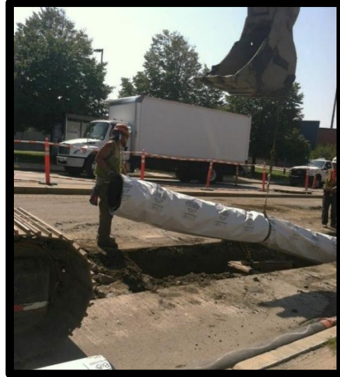
Installing Water Main Albany Street
