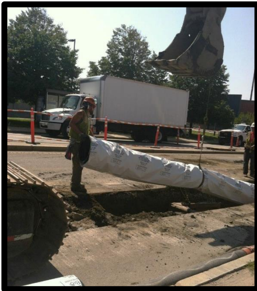
Installing Water Main Albany Street
