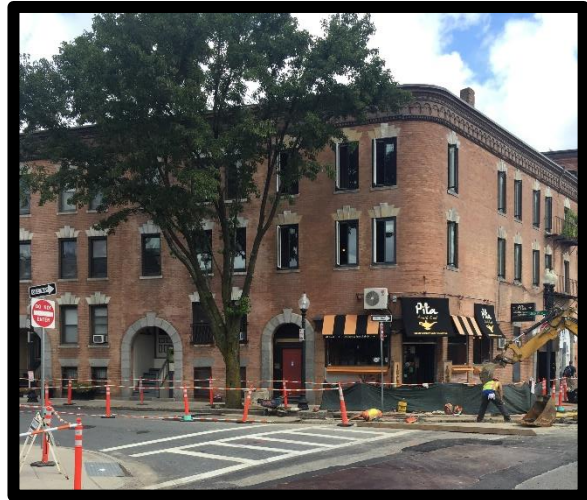
Preparing Water Tie-In Albany Street at Union Park Street
