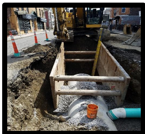
Dudley Street Installation of 48" Drain Pipe
