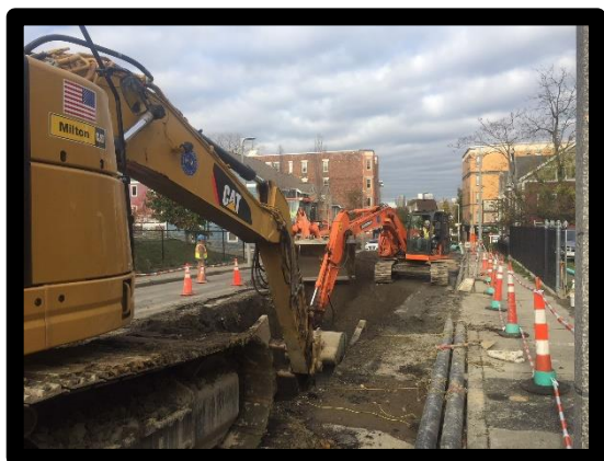
Dudley Street Excavation for 24" Sewer Installation
