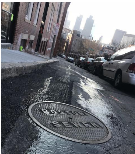
Sewer Manhole Snow Hill Street
