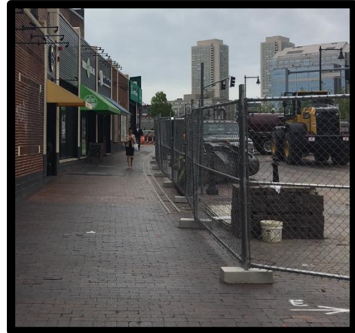
Fenced in Work Zone - Typical Cross Street
