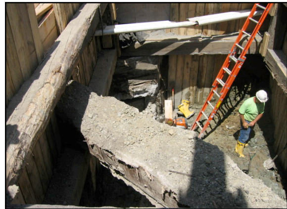
Installation of Special Manhole at Farragut Rd. and East Second St.
