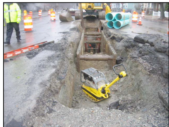
Installation of 18" sewer on Farragut Road.
