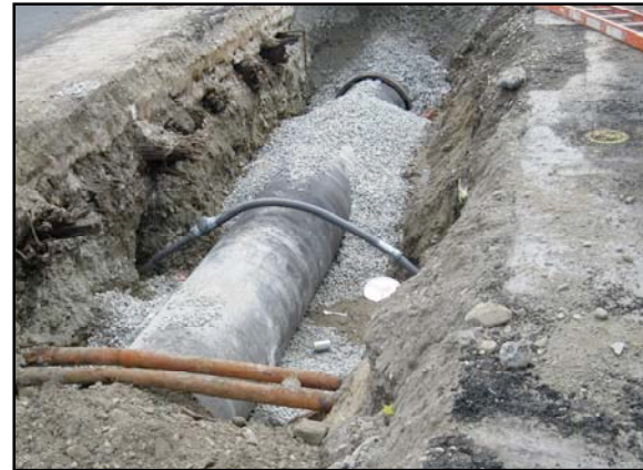
Installation of 24" drain on East Fourth Street.
