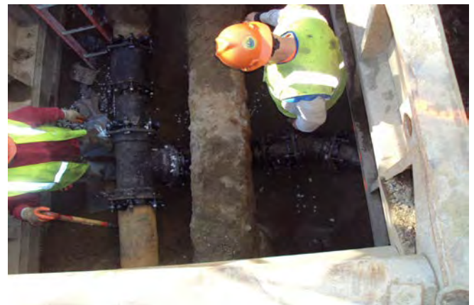
Water main construction at I Street and East Second Street
