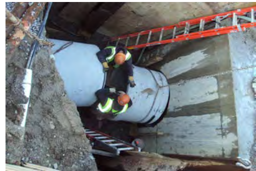
48-inch storm drain construction at Outfall 078
