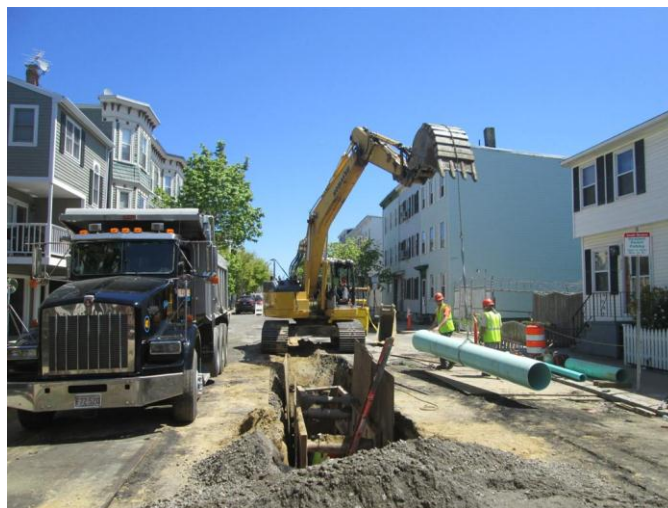
Installation of 18" sewer between I Street and Emmet Street
