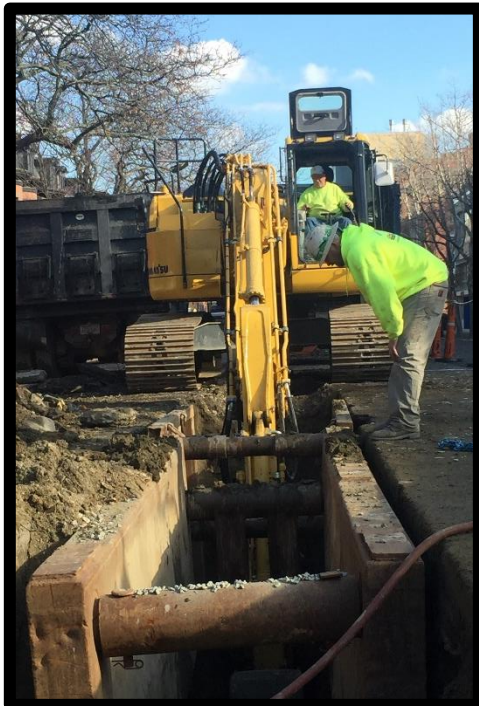
Sewer Main Installation Warren Avenue
