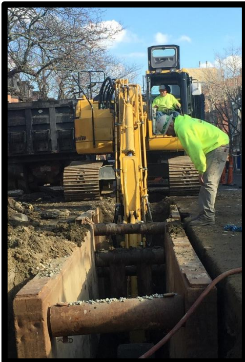
Sewer Main Installation Warren Avenue
