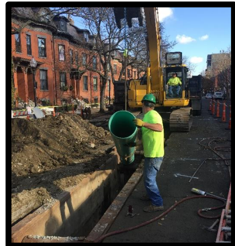
Sewer Main Installation Warren Avenue near Dartmouth Street
