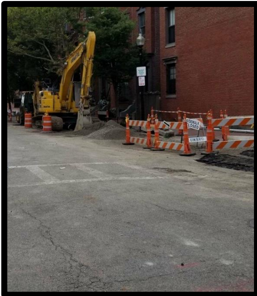
Securing Work Zone and Pedestrian Access Shawmut Avenue
