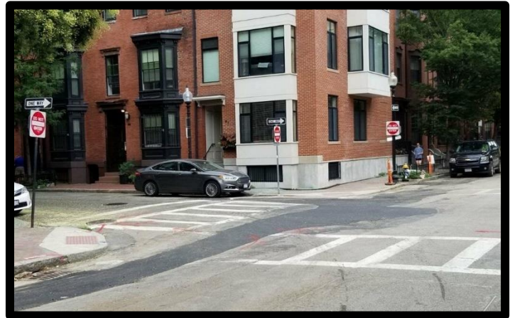
Temporary Pavement Shawmut Avenue at West Springfield Street
