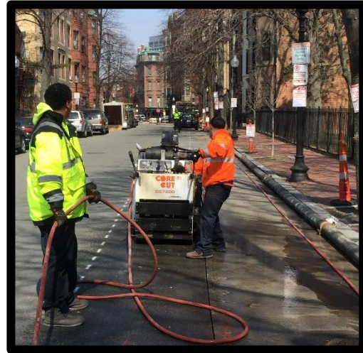
Saw Cutting Water Trench Typical Set Up
