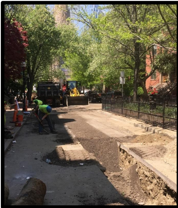
Backfilling Water Trench Rutland Square
