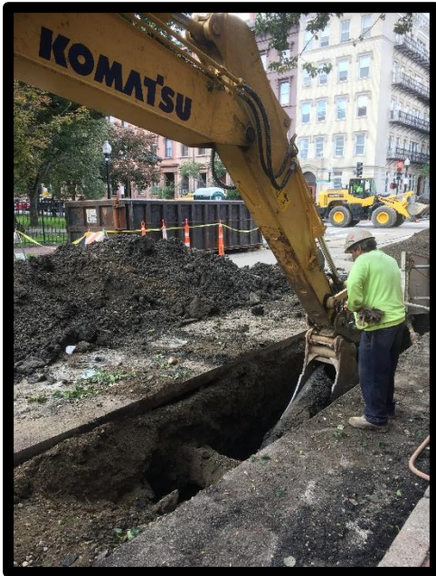
Water Main Installation Shawmut Avenue At Blackstone Square
