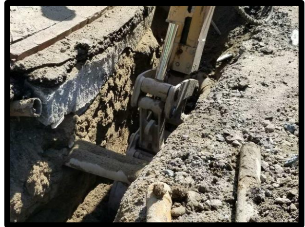
Excavating Around Utilities Shawmut Avenue
