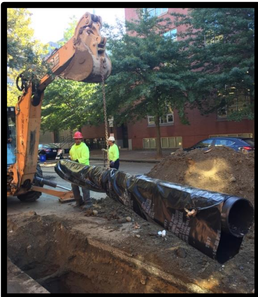
Water Main Installation Warren Avenue
