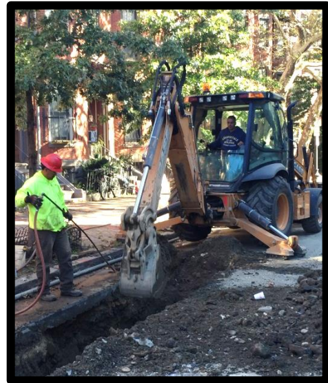
Water Main Installation Warren Avenue
