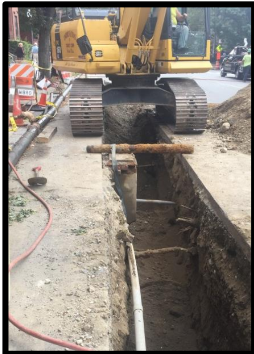
Water Main Installation Warren Avenue
