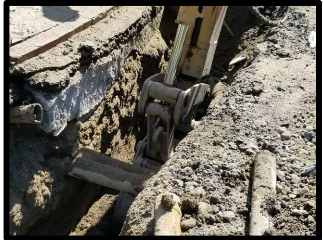
Excavating Around Utilities Shawmut Avenue
