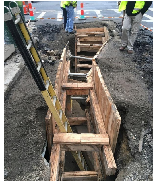
Phase II Excavation
