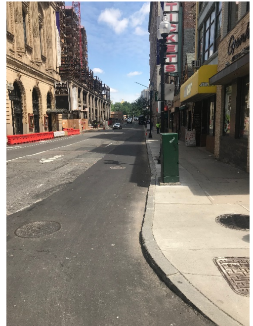
Restored Trench & Sidewalk
