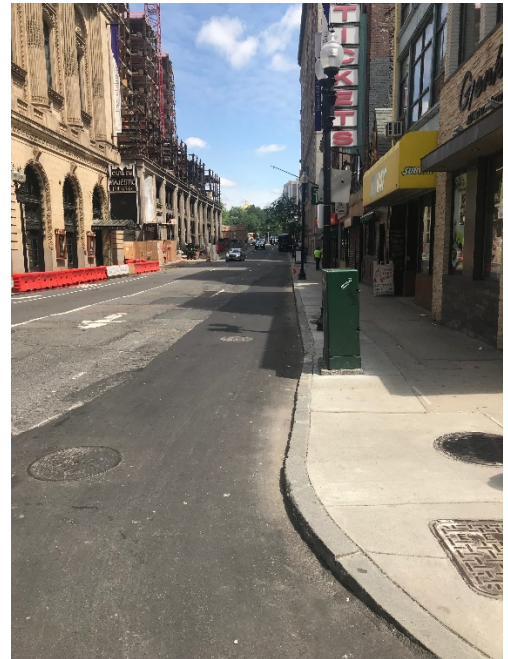
Restored Trench & Sidewalk
