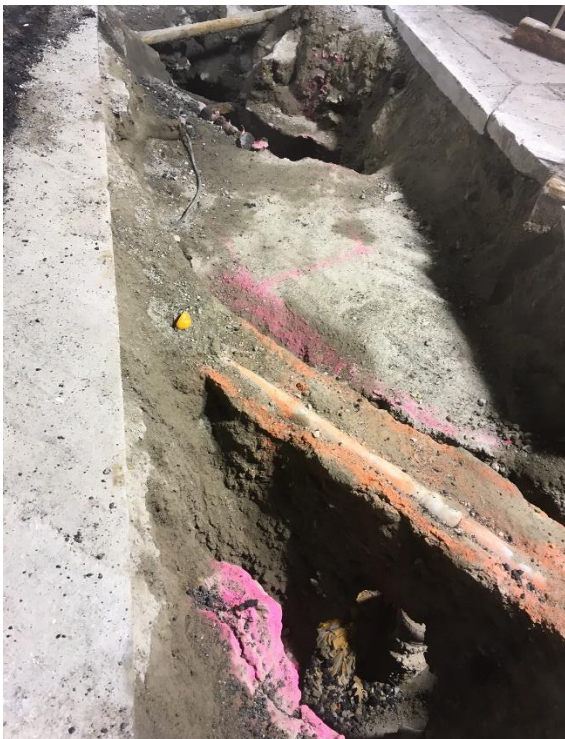
Sewer Replacement Excavation (multiple utilities above sewer)
