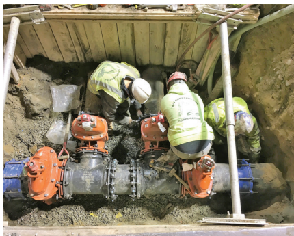
Installing water meters on Brookline Avenue.
