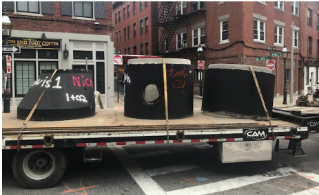
Catch Basins ready for installation
