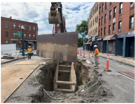
DUDLEY STREET INSTALLATION OF 24" SANITARY SEWER
