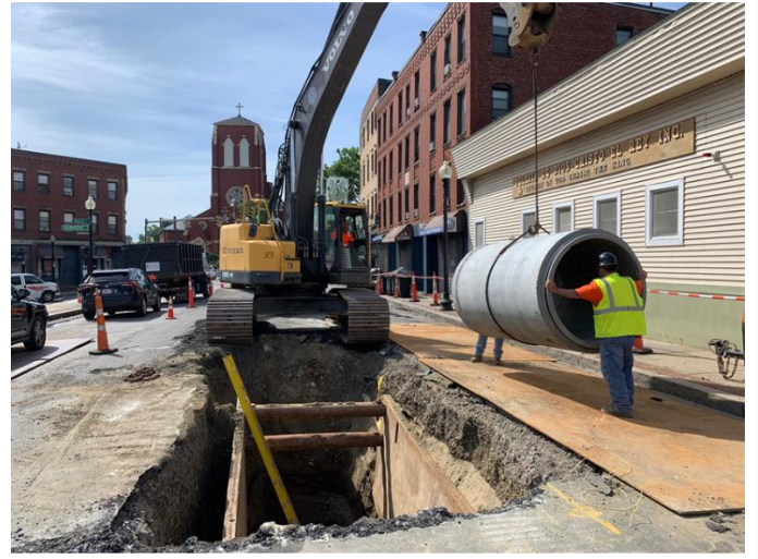
DUDLEY STREET INSTALLATION OF 48" STORM DRAIN
