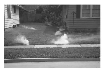
Residents of Mattapan please be advised CDM Smith and Martinez Couch & Associates contractors for Boston Water and Sewer Commission (BWSC) will be smoke testing sewers to locate sources of storm water inflow entering the sanitary sewer system. Smoke testing will enable BWSC to locate direct and indirect connections from sources such as catch basins, roof drains, and broken sewer pipes.
