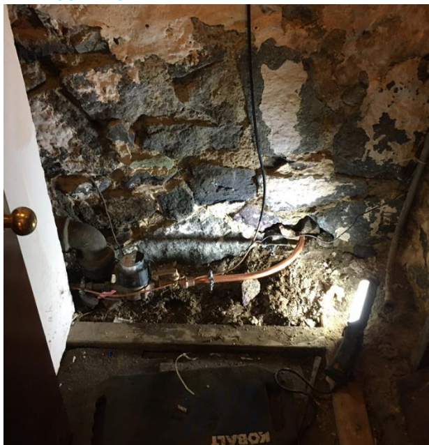
Copper Pipe Connected Water Meter
