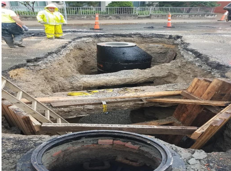
Contract 20-309-012 SOUTH BOSTON SEPARATION Installation of Drain Manhole - West Fourth St at Dorchester Ave
