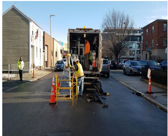
Set up for Combined Sewer Cleaning on B Street
