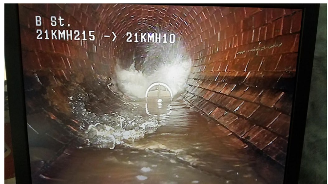
Pipe Cleaning B Street
