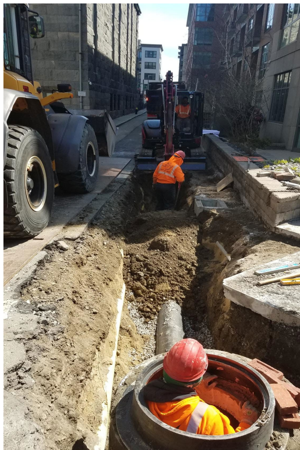
Drain line installation on Silver Street from Dorchester Avenue
