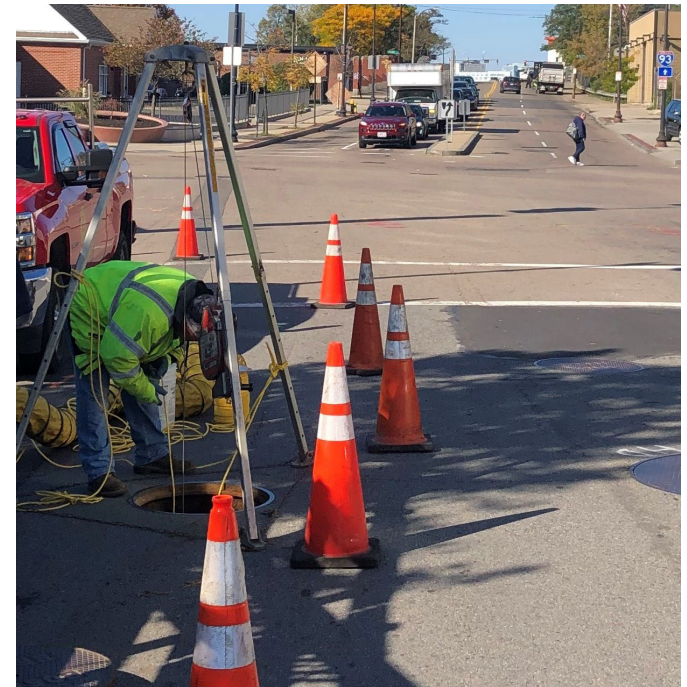
Inspection of Manhole "D"
