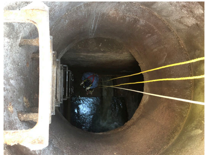
Inspection of Manhole "B"
