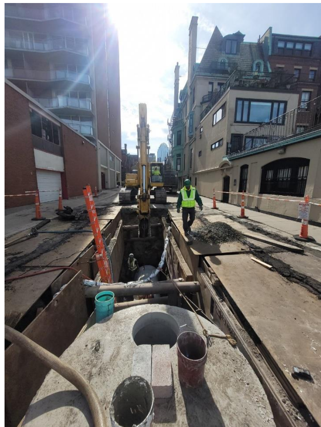
Contract 20-308-005 36" RCP replacing a 3'x4' wood stave
