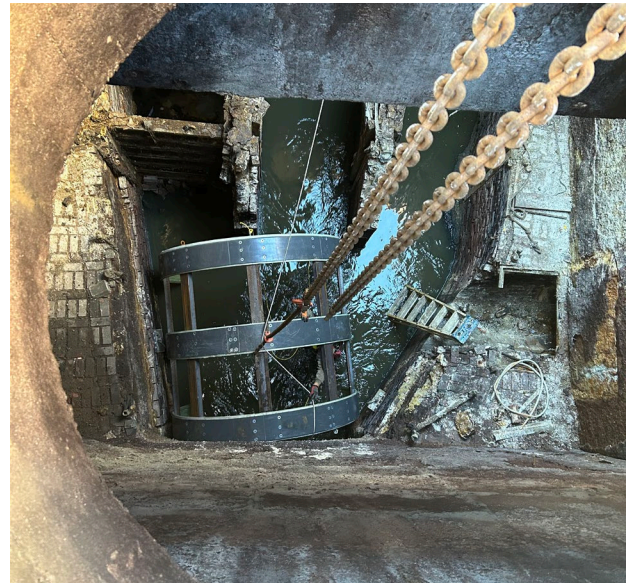
Mandrel pull in Special Manhole D
