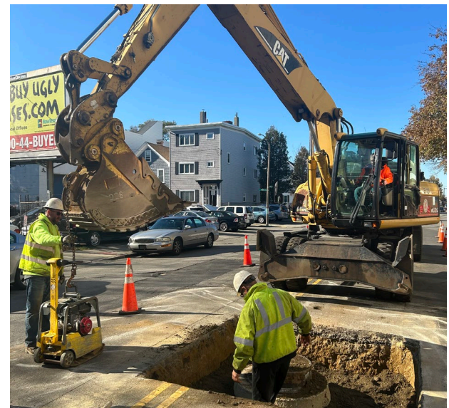
Preparing to receive the mandrel on Preble Street
