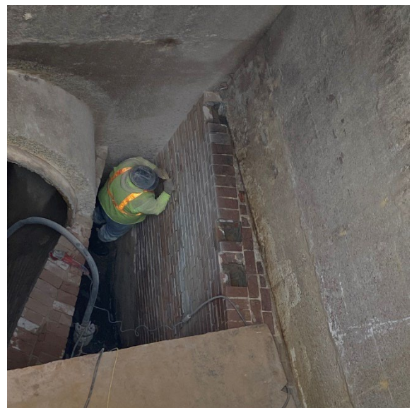
Refurbishing brickwork in Special Manhole E
