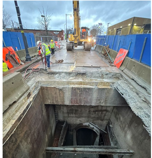
Inside the work zone on Southamptom Street
