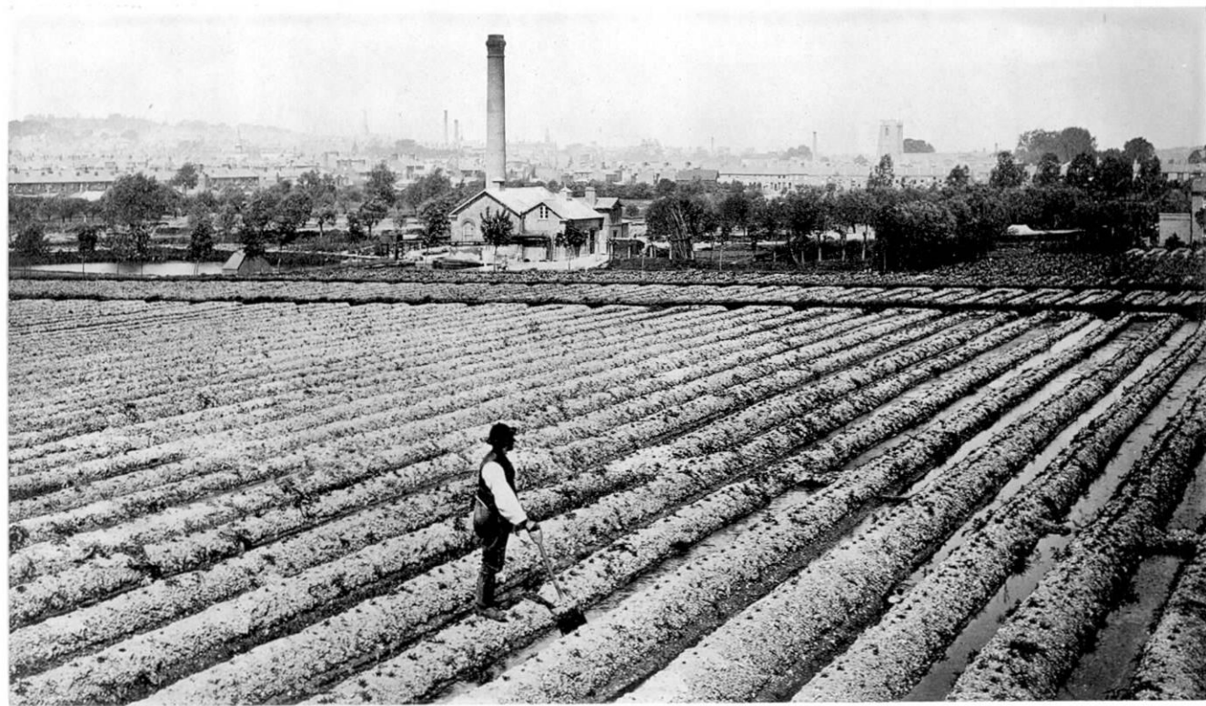
Luton, England. View at sewage filtration fields, 1885.
