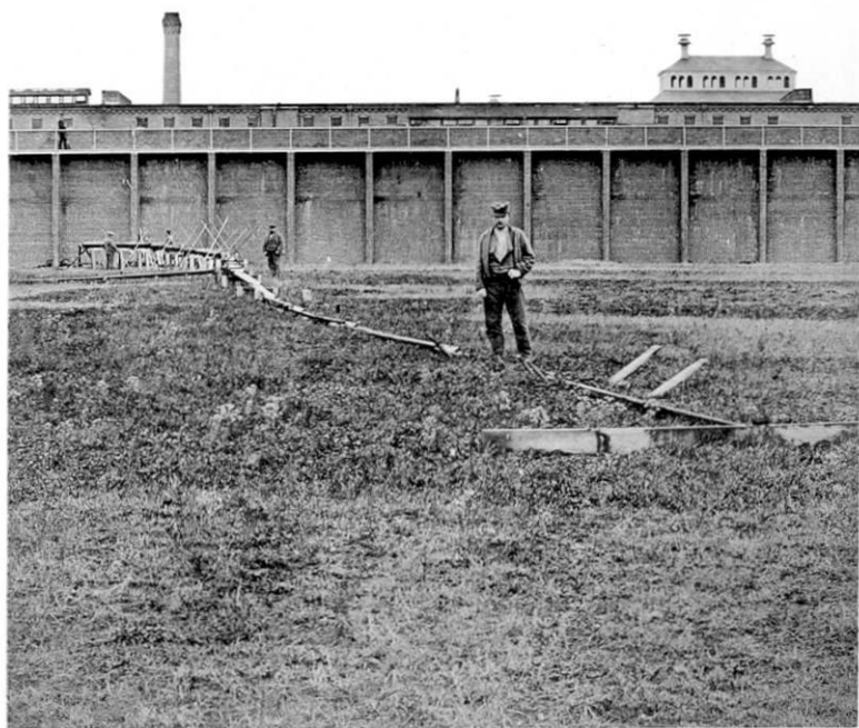
Sewage disposal at State Prison, Concord, Mass., 1884.
