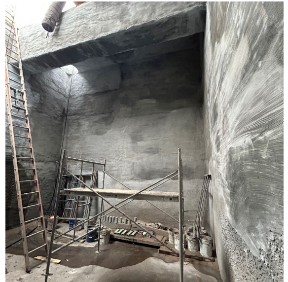
Inside Special Manhole E after cement-based lining work
