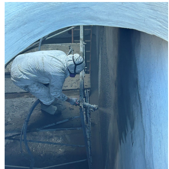
Crews apply cement-based spray-on liner
