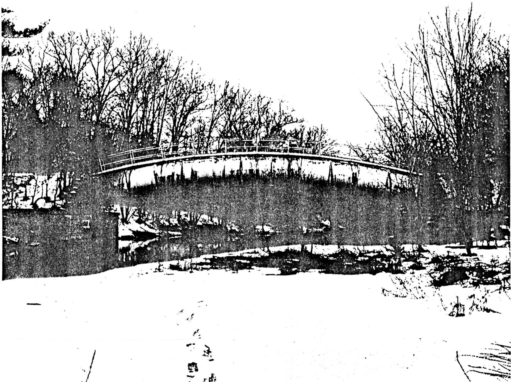
Pipe Arch on the Sudbury River Siphon, Weston Aqueduct, Framingham and Wayland. Built 1902-1903.
