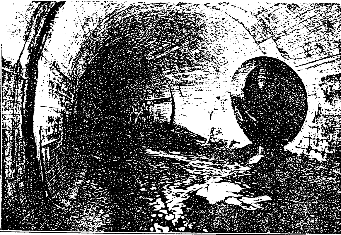
JUNCTION MAIN CHANNEL STONY BROOK AND BUSSEY BROOK BRANCH CONDUIT AT REDUCER ON MAIN CHANNEL AT FOREST HILLS SQUARE.
