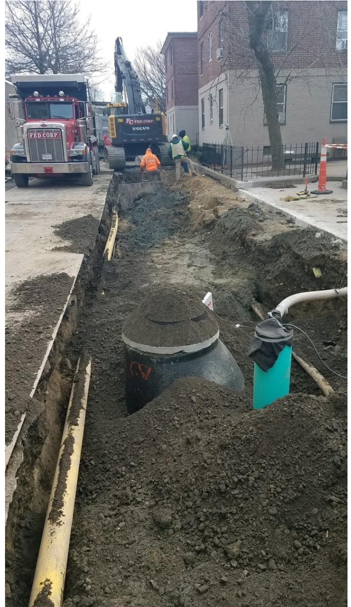
Crews work on drain trenches along Flaherty Way
