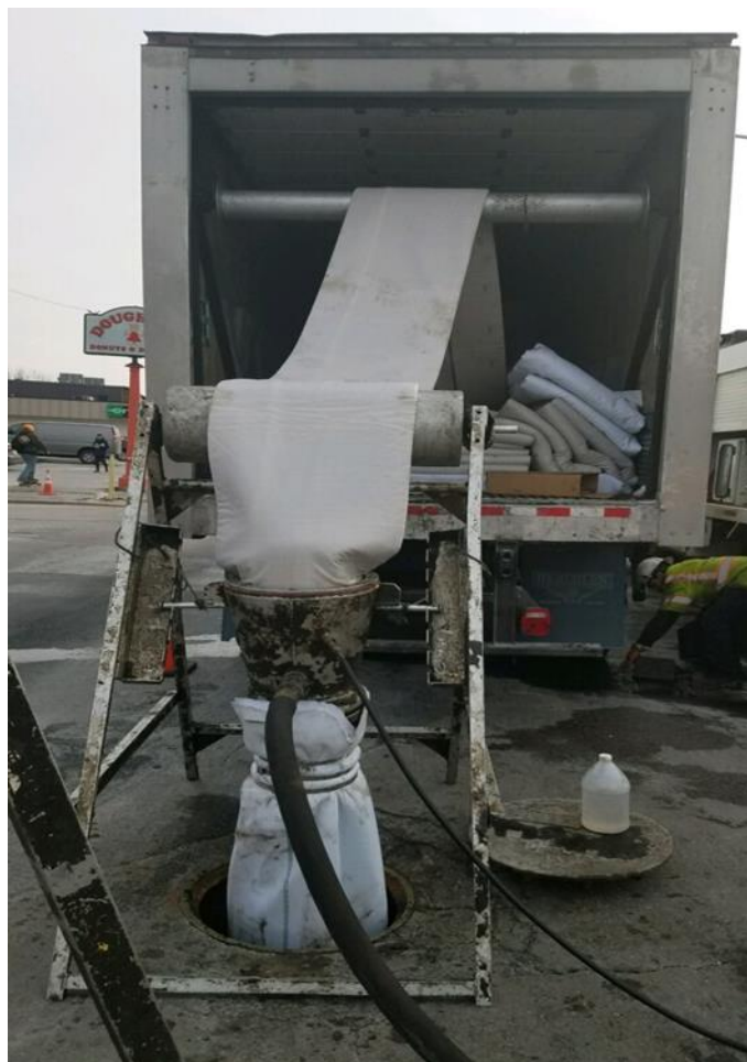
Installation of 15-inch structural liner on Dorchester Avenue at A Street.
