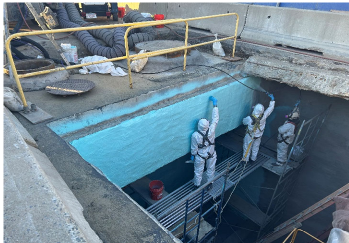
Crews apply spray-on liner and epoxy in MH E.
