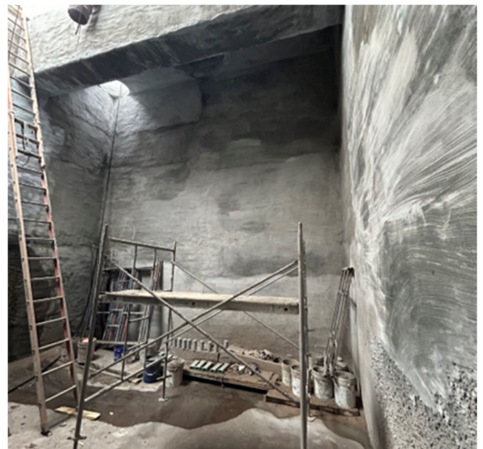
Inside Special Manhole E after cement-based lining work
