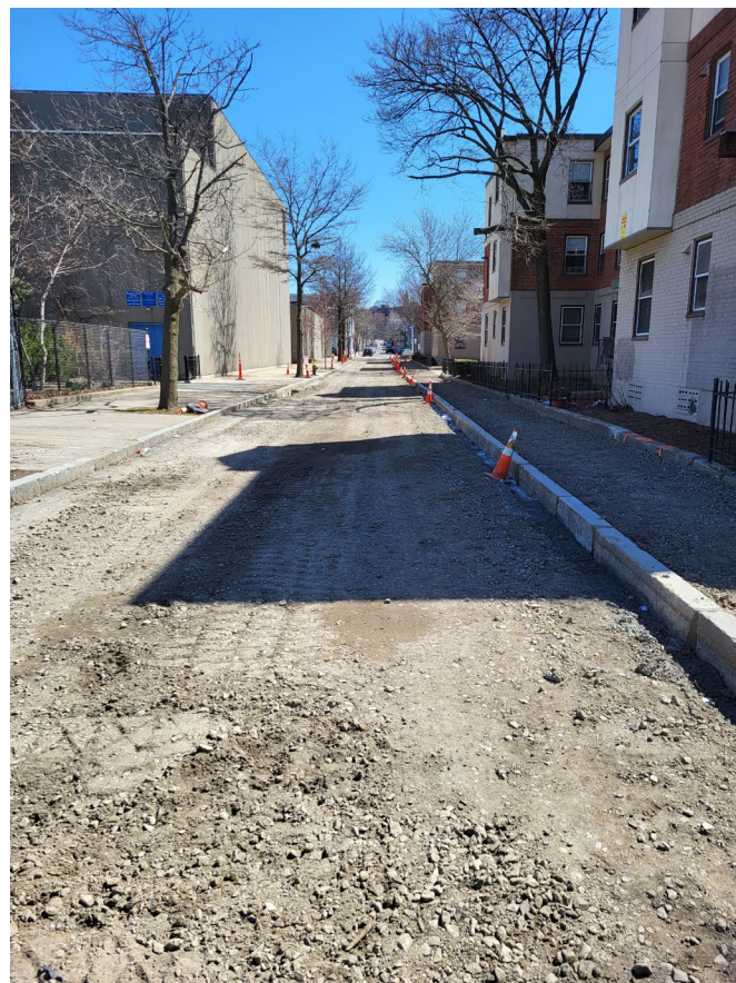
Preparation for temporary paving and sidewalk placement on Orton Marotta Way.
