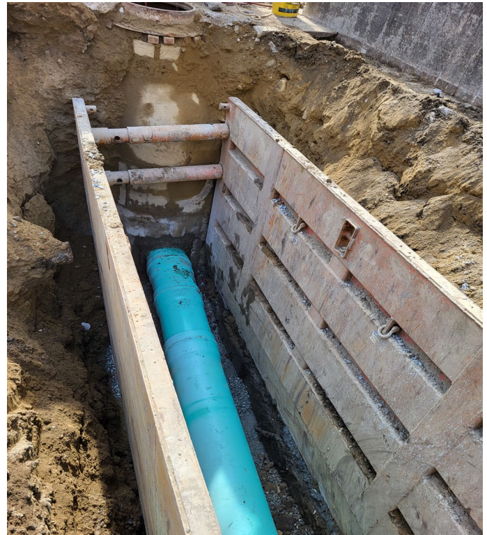
18-inch PVC Drain Orton Marotta Way
