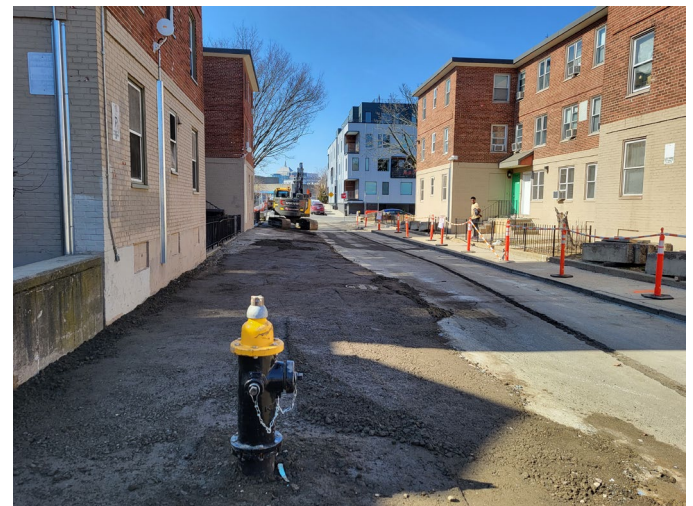
New hydrant Orton Marotta Way
