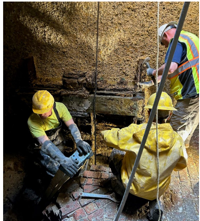
Crews remove old gate in Special Manhole C.
