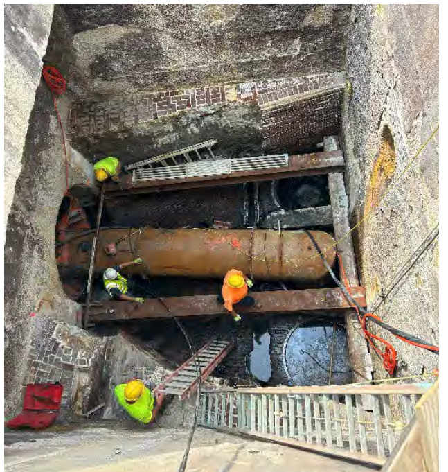
Slipline guide beams and bypass in MH D
