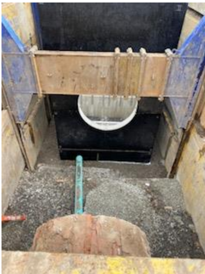
Talbot Ave/ Harambee Park - De-Nitrification Vault/Chamber. Green Infrastructure Pilot Project
