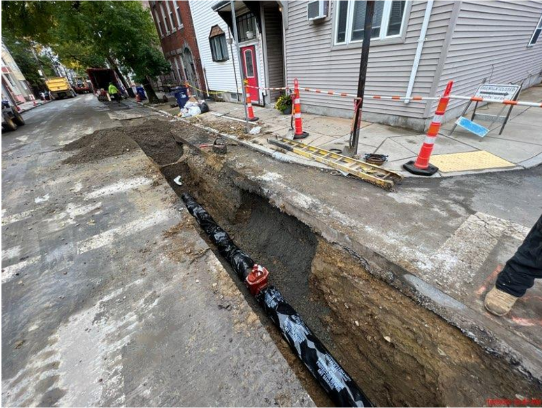
Cottage St – 8-inch ductile iron, zinc coated class 56 pipe with 8-inch gate valve. Poly wrapped with V-Bio Polyethylene Encasement to inhibit corrosion.
